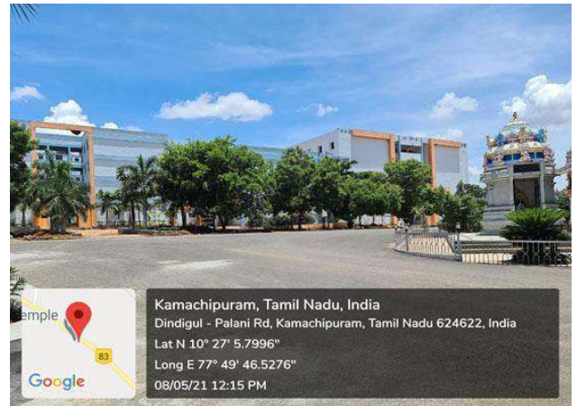
Fig. 10.2: View of all Buildings
